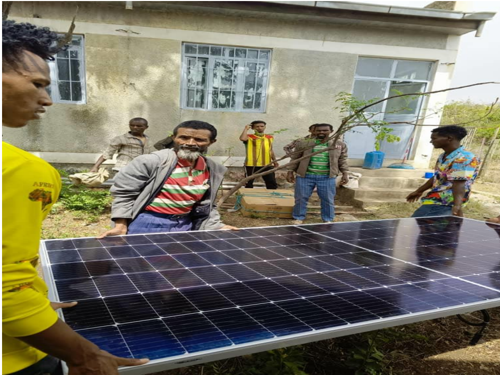
Figure 1: Logistics During Installation
