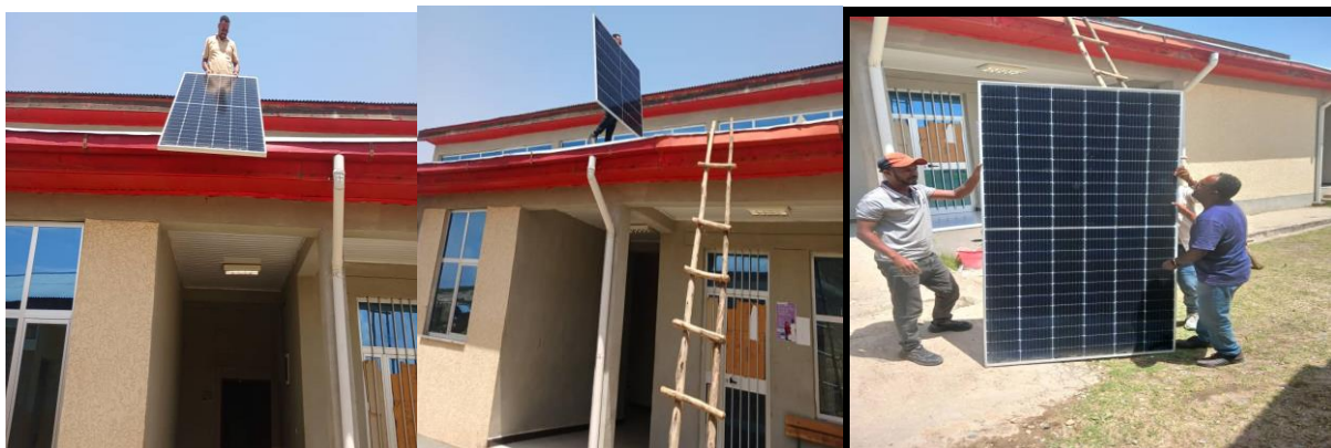
Figure 3: Pre-assembly of Solar PV at Agazi Health Center
