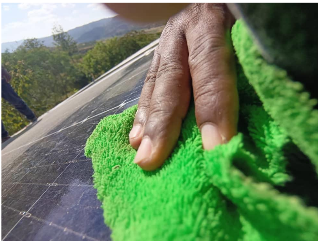
Figure 2: Solar PV Cleaning procedure as preventive maintenance
