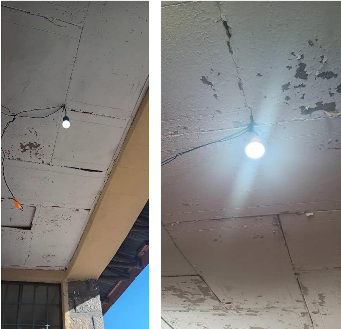
Figure 11: Lighting Service after Installation of Mitslsl Afras health post
