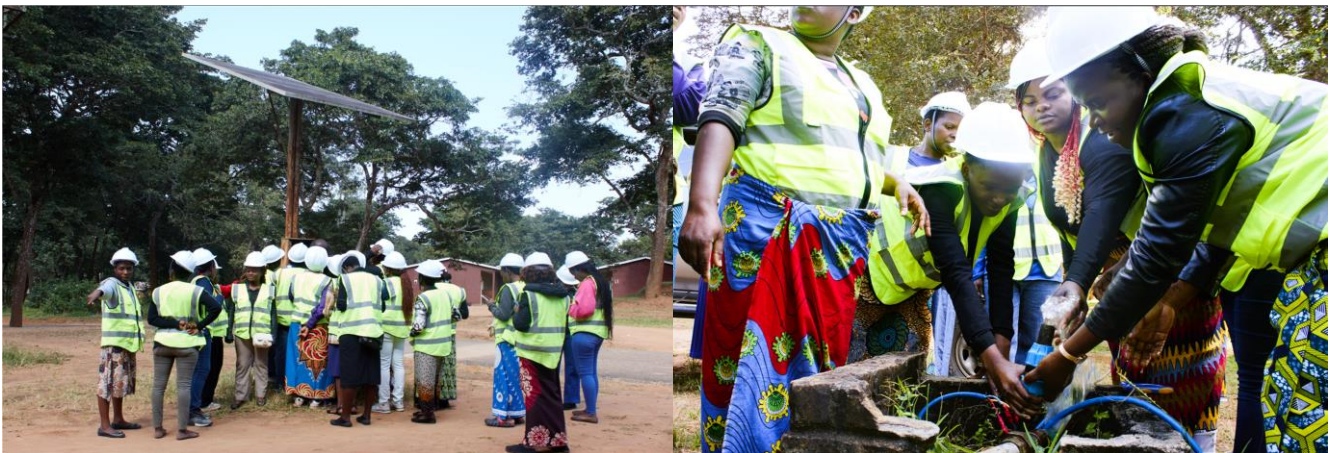
Figure 4: Participants Installing a solar water pump on campus
