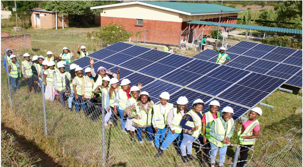
Figure 5: Site Visit at Choma health facility Solar PV Plant
