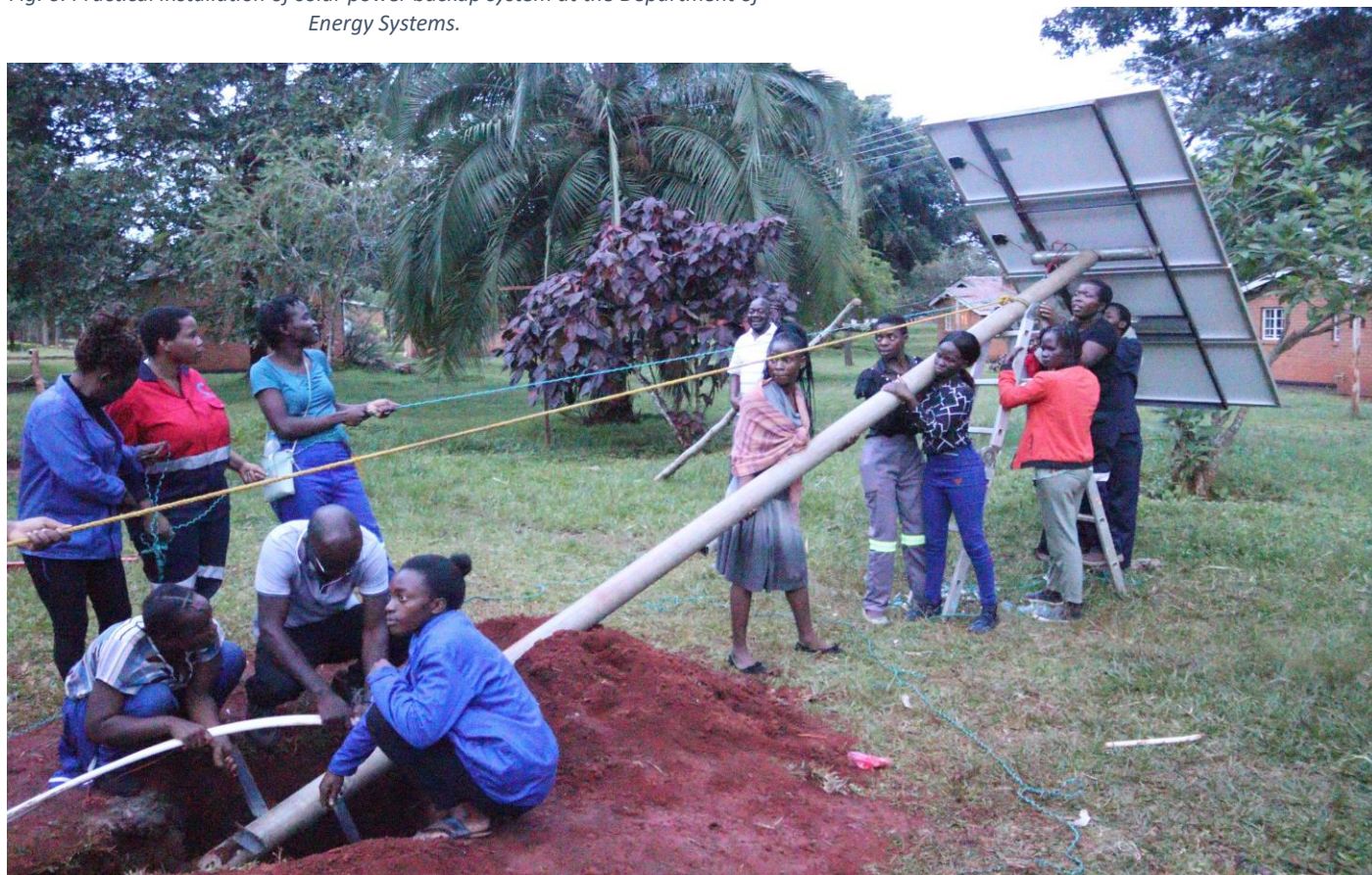
Fig. 7: Practical installation of the pole mounted solar PV system
